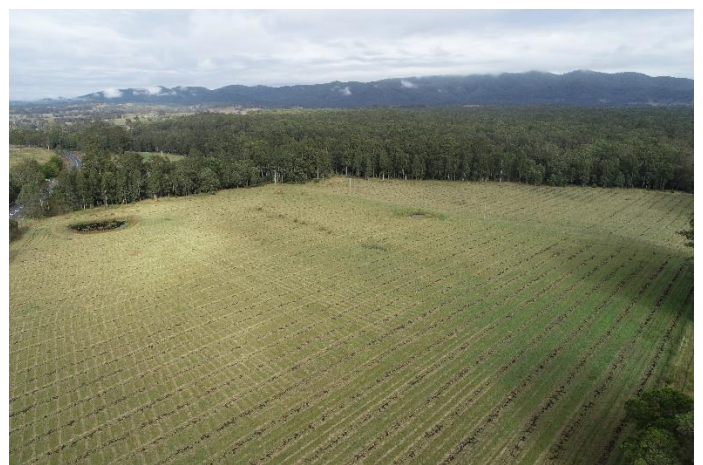
Plate 2: Ground preparation of Offset Area 4 – Rodgeron 2021.
